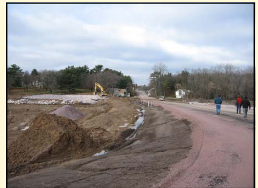
Rebuilding of STH A embankment.
